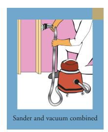
Sanding would be effective only if the mold is limited to the surface of the wood. Wood that is decayed should be replaced. Vacuum up all the mold and sanding debris.
